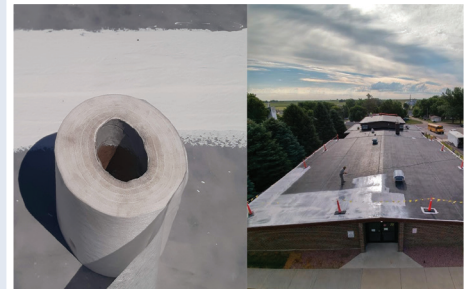
Apply 2 part epoxy primer, then reinforce seams and details using polyester mesh
