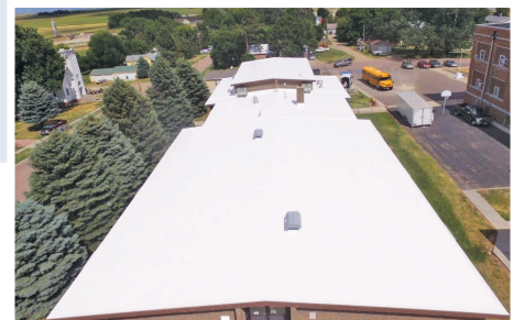
The finished roof
