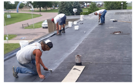
Repair EPDM saturated/delaminated areas
