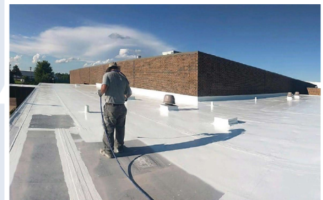
100% Silicone Top coat application
